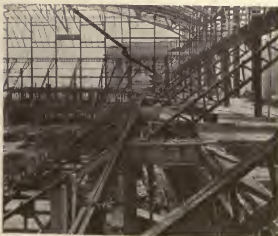
A SECTION OF THE BALCONY STEELWORK
